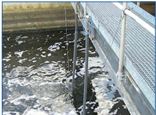
ammo::lyser mounted on railing
