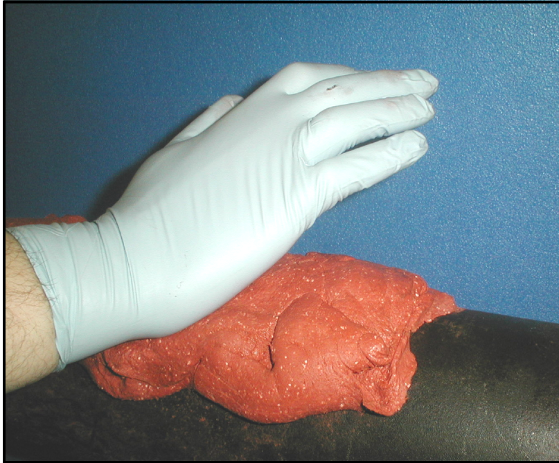
Figure 8: Applying DMP-3 Damping Material
